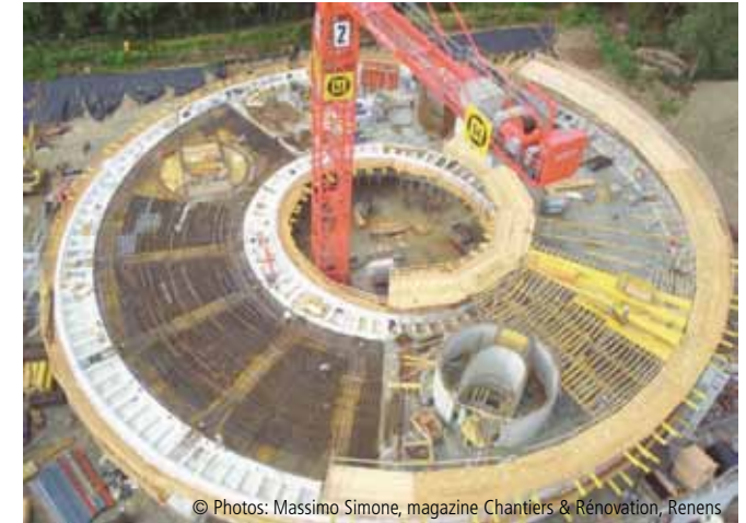
© Photos: Massimo Simone, magazine Chantiers & Rénovation, Renens
