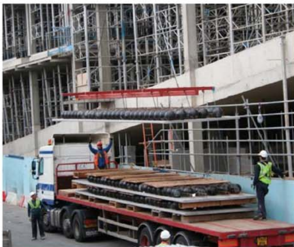
Heavy lifting: The precast concrete "biscuit" base
