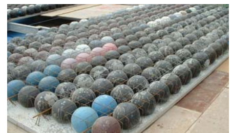
top left A model showing how Sheffield University's Learning Resource Centre will look when finished above The Cobiaxdeck system as it appears when delivered to site left Construction under way on the Sheffield University project
