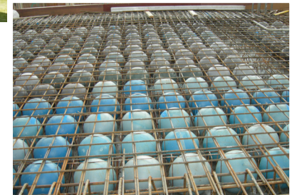
CobiX void formers are directly placed into the semi pre-cast elements during fabrication.
