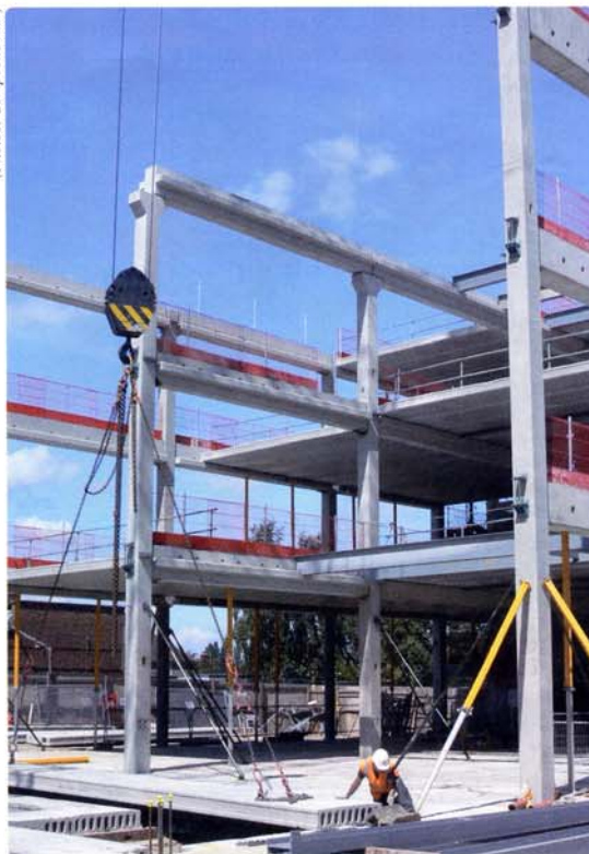
Figure 1: Frame construction during Phase 1 at Chessington Community College.
