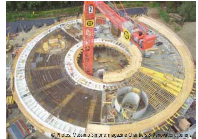
© Photos: Massimo Simone, magazine Chantiers & Rénovation, Renens
